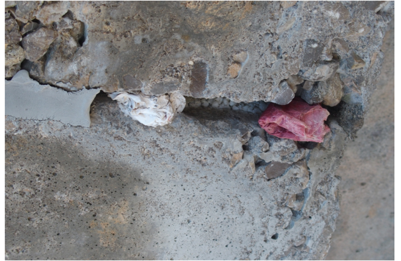
Hidden in the wall (A. Mietzner 2017)
