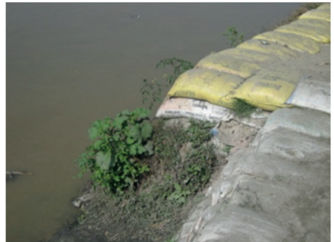
Figure 20. Sandbagging of river bank, Manohara squatter settlement.
