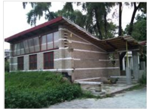
Figure 3. The completed prototype climate responsive school building at the premises of IoE.
